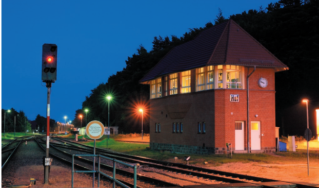
Fig. 1-13: Dispatcher signal box and main light signal (left)
