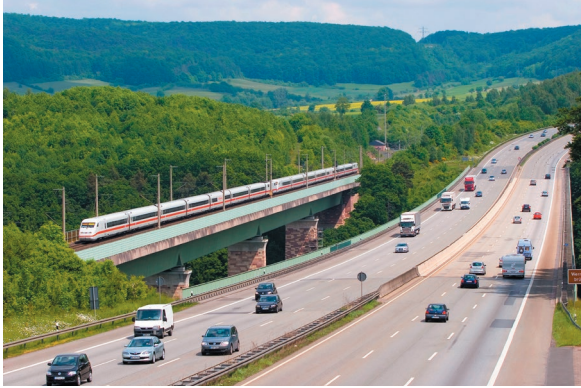
Fig. 1-9: A double railway track has the same capacity as a six-lane motorway. Photo: DB AG/Bartłomiej Banaszak
